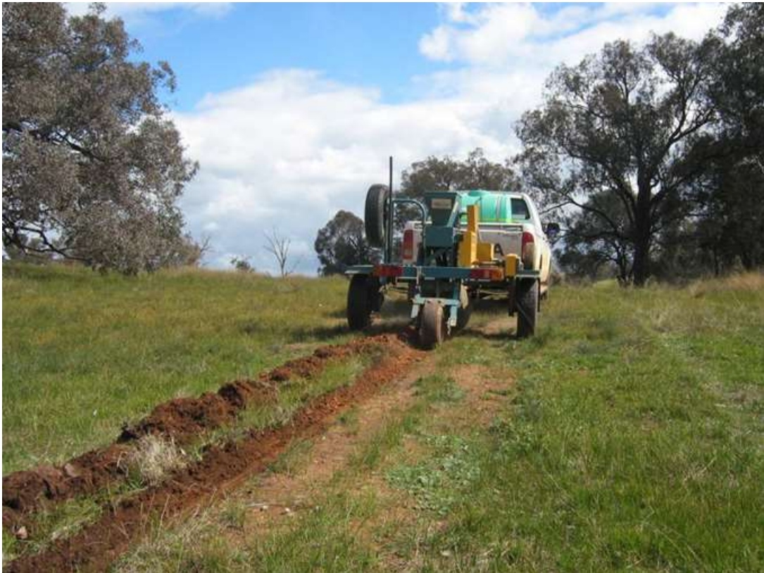
Figure 9 – Mechanical direct-seeding occurring at Woomargama (Photo by Nigel Jones)
